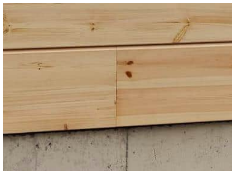
Photo: Seam on log connection point (© Kontio)
