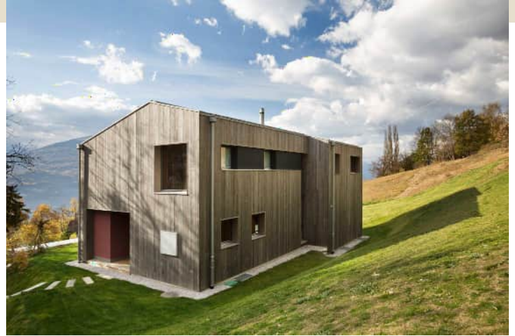
Photo: facade cladding on log wall, private house in Switzerland (© Kontio)
