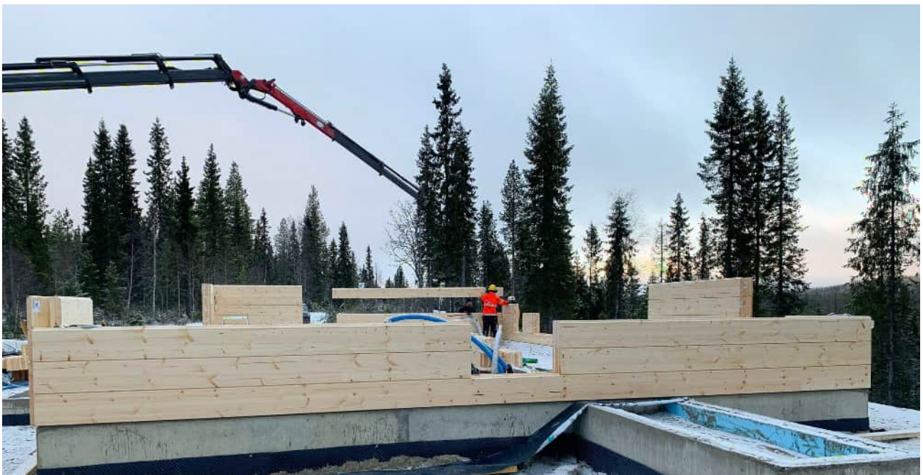
Photo: Construction of log frame (© Kontio)
